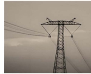
Fig. 4. Aerial images of straight electric power towers.
