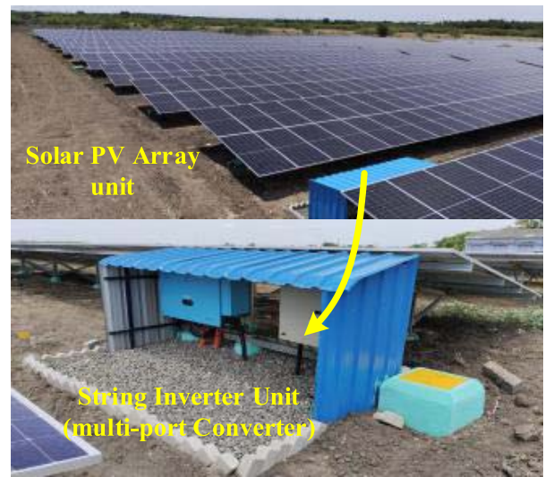
Fig. 12. Implementation of proposed multi-port DC-DC converter for DMPPT operation in real time solar PV plant.
